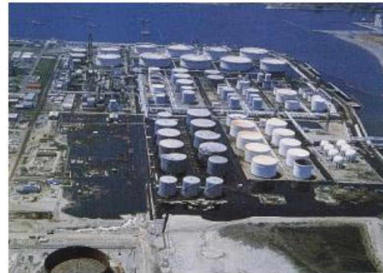
Figure 9. Spilled oil inundated a refinery area in Sendai at the 1978 Miyagi Earthquake (Courtesy of Kahoku Simpo Publishing Co.)
