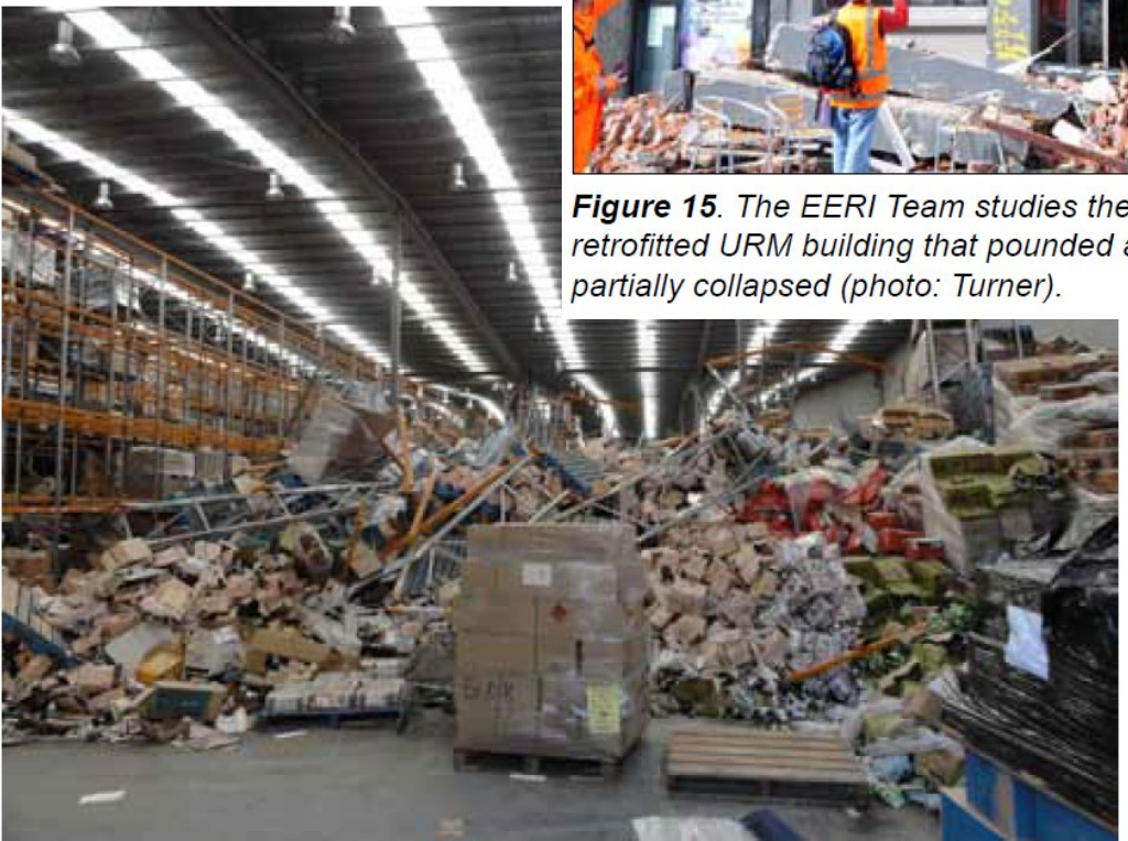
Figure 18. Collapse of storage racks (photo: Elwood).
