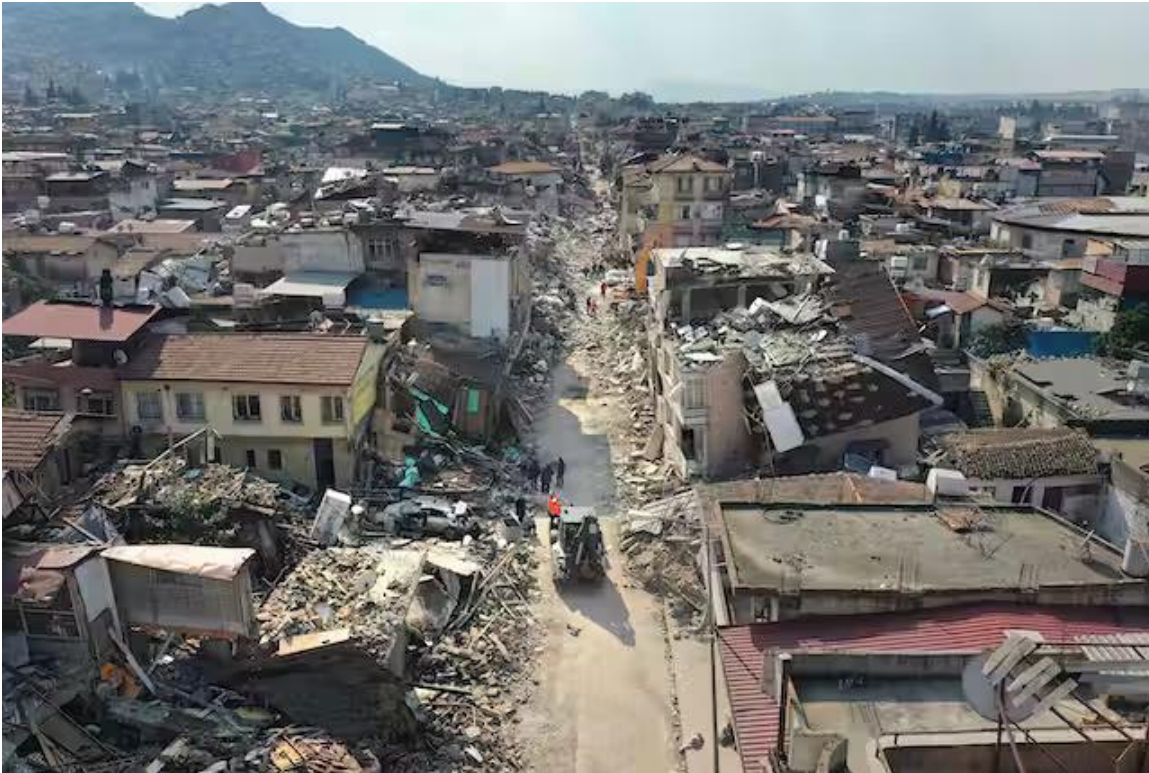
Figure 2. Examples of damage in the city of Antakya after the February 6 th Gaziantep Mw 7.8 earthquake. The city of Antakya is built on young sediments with a shallow water table similar to the geologic setting found in the Mississippi embayment (courtesy AFAD, Turkey).
