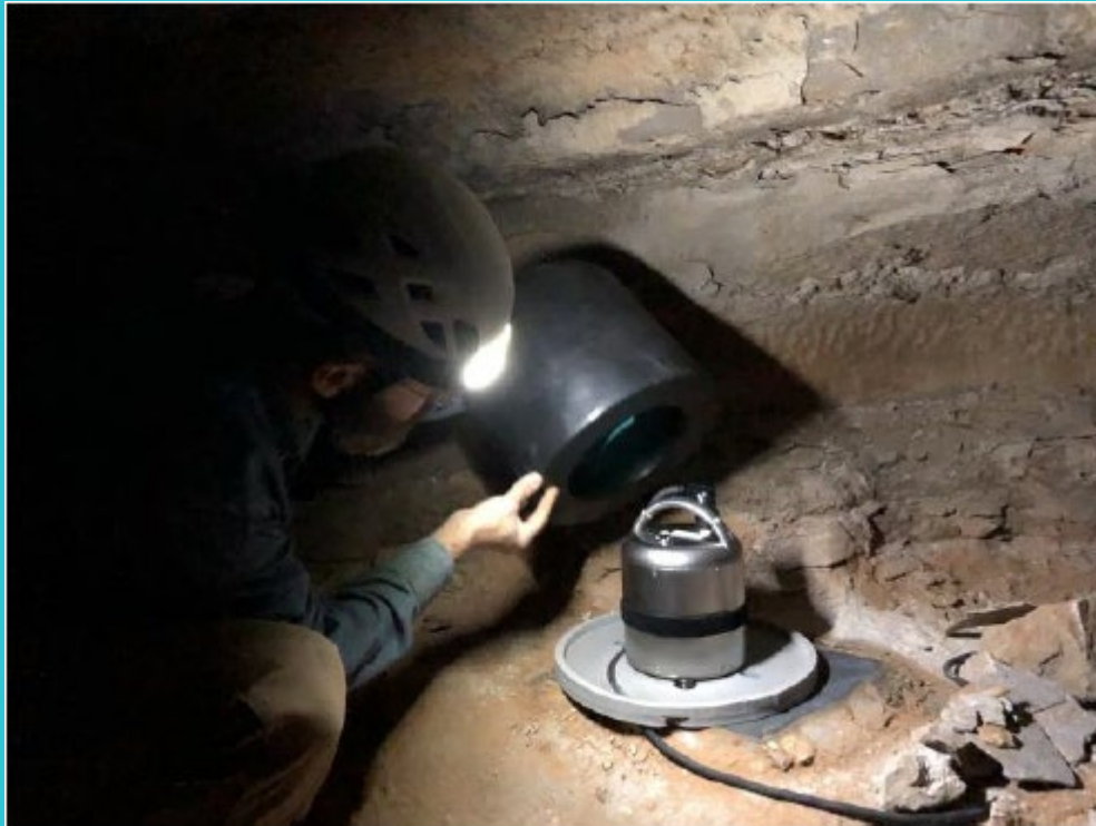
Tennessee Cave - Underground installation
