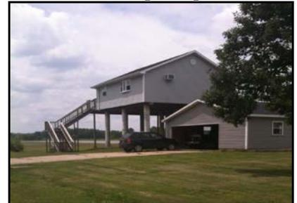
The elevation method is dependent on the structure's condition, flood hazard, local floodplain regulations, and owner's financial condition. When elevating, it is essential for all utilities (air conditioner, water heater, furnace, etc.) to be elevated to or above the Base Flood Elevation.
