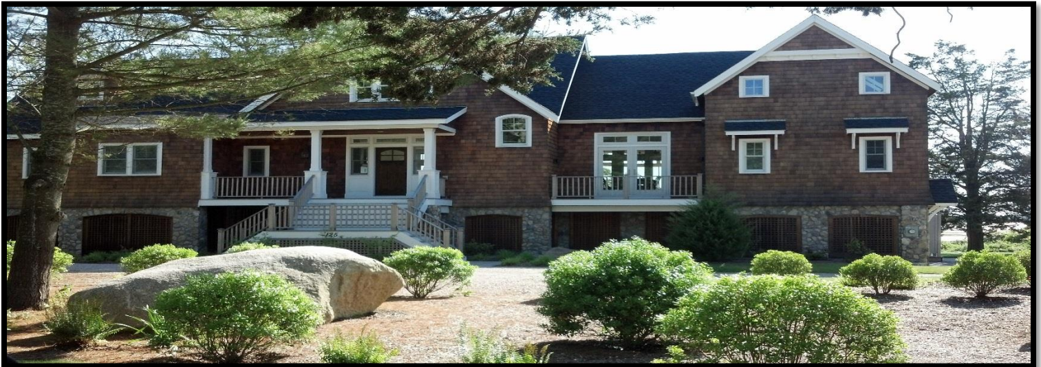
An elevated home above the base flood elevation (BFE) in Rhode Island. Photo credit: Association of State Floodplain Managers
