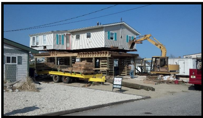
Home elevation is one technique to protect against future flood damage and loss. Photo credit: Association of State Floodplain Managers
